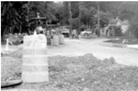
Infrastructure Street Repairs
