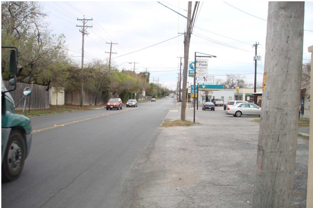
Figure 1 Pedestrian routes are not defined or inconsistently routed and lack basic pedestrian amenities.
